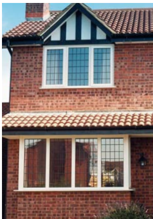
Casement window with imitation sash horns
